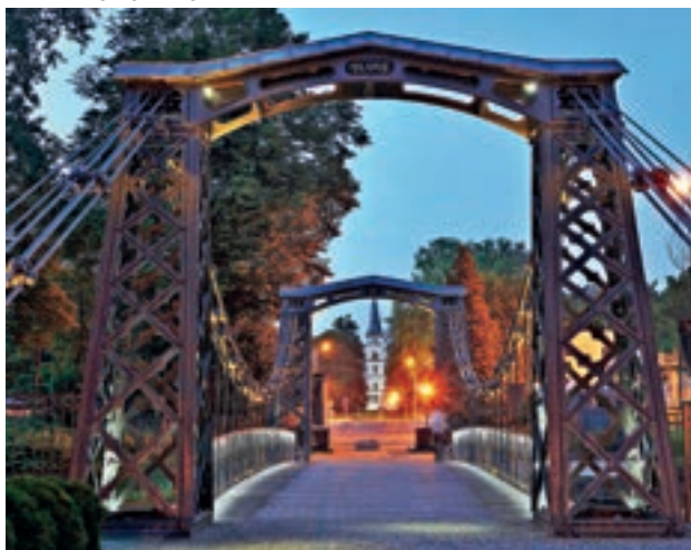
Iron hanging bridge in Ozimek
